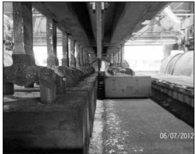
Figure 3. Anodes placed carefully in cell on resistor bed.
