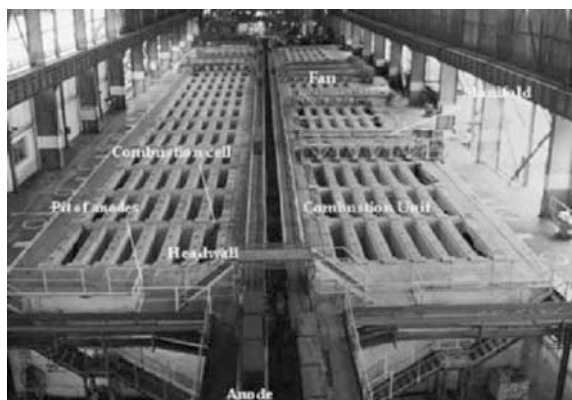
Fig 1. Anode baking furnace building overview.
