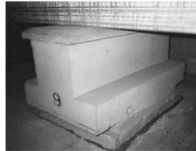
Figure – New Cross-Over Busbar Support in Place
