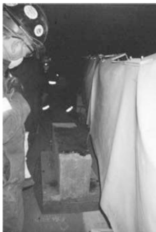
Figure – Work Inside the Tunnels
