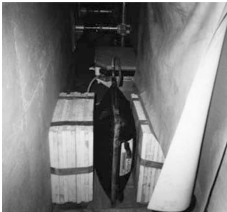
c) Pulling the Old Support along Tunnel Alley
