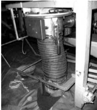
Figure 4 Flexible exhaust leg with dual flap damper
