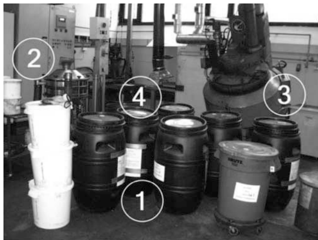
Figure 1: 1) Part of aggregate inventory; 2) Multideck screening machine; 3) Mixer Eirich RV08; 4) Vacuum vibroformer.
