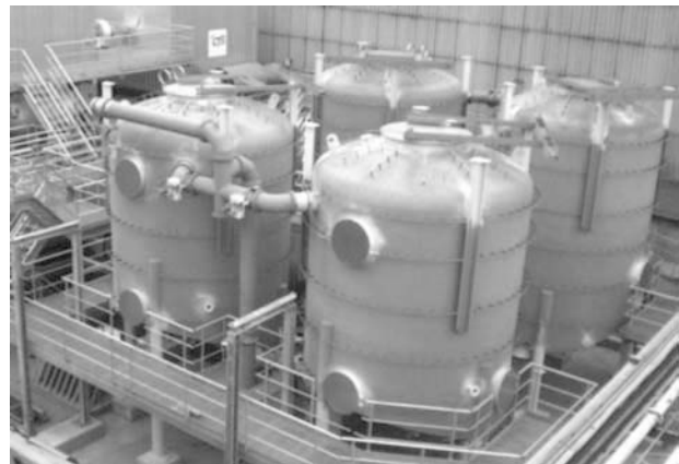
Figure 5: Pre-filter System of a FTS (during installation)
