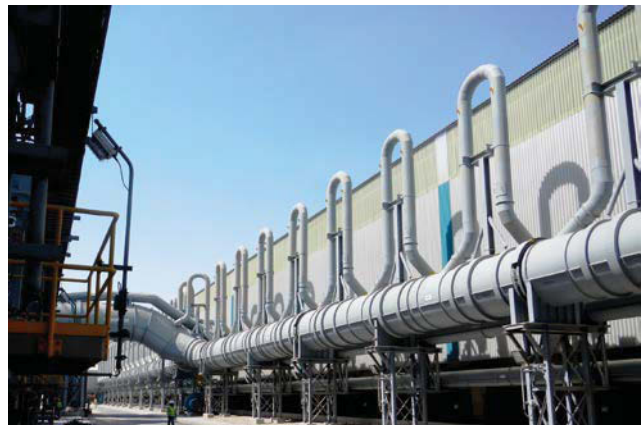
Figure 2: Hairpin coolers on Ma'aden GTC1.
