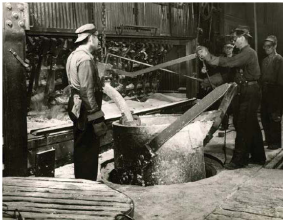
Figure 2. Siphoning aluminum metal from a HS Söderberg cell at the Alcan Arvida smelter in 1944. Source; Rio Tinto Alcan
