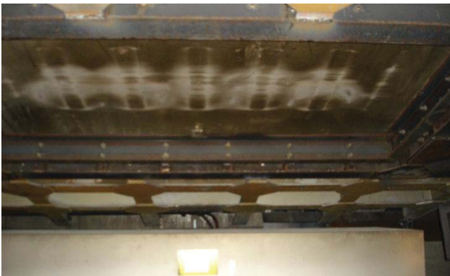
Fig. 9: Pole marks on stainless steel window reveal details of internal stirrer structure.
