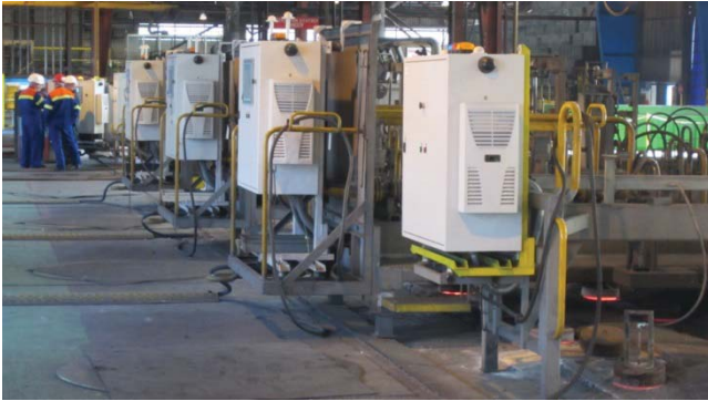
Figure 4: Demonstration fire at Saint Jean de Maurienne
