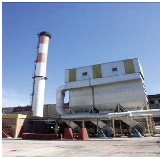
Figure 1: Former Fume Treatment Centre at Aluar
