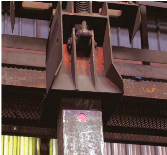
Figure 3: RFID-tag installed in aluminium anode rod (retrofit) just below bell, in its final shape.
