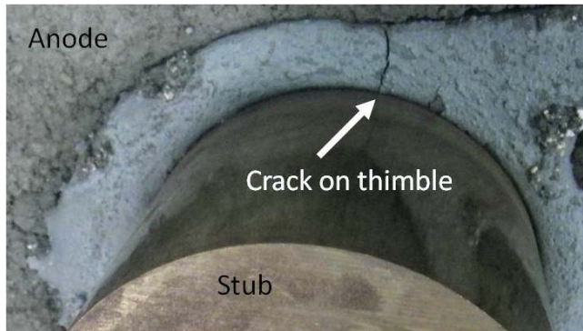
Figure 14. Validation of the predicted equivalent plastic strain based on a crack observed in an industrial thimble.
