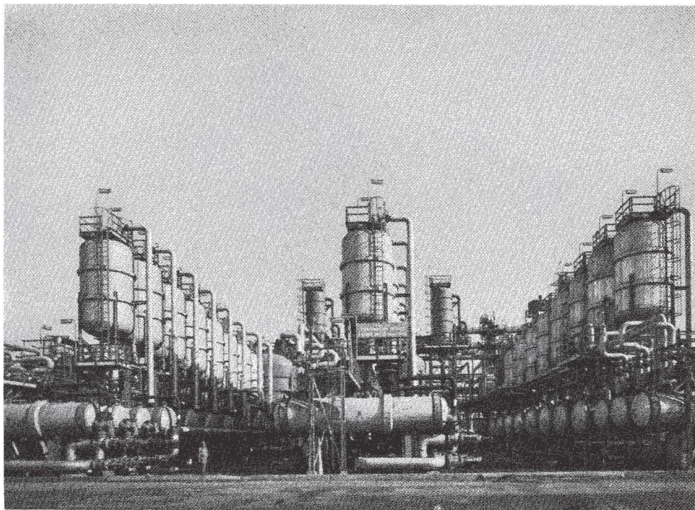
Figure 6 - Heat economy systems in a sodium aluminate evaporation plant in Sardinia. Shown are three lines of 9 flash evaporators each with preheaters. Evaporation capacity of 3 x 90 tons/hour. (Courtesy Escher Wyss Co.).
