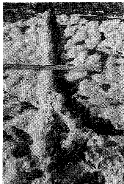
Figure 24. Erosive enlargement of bottom heave cracks in cathode is similar to pot hole formation mechanism. Pot life was 501 days.
