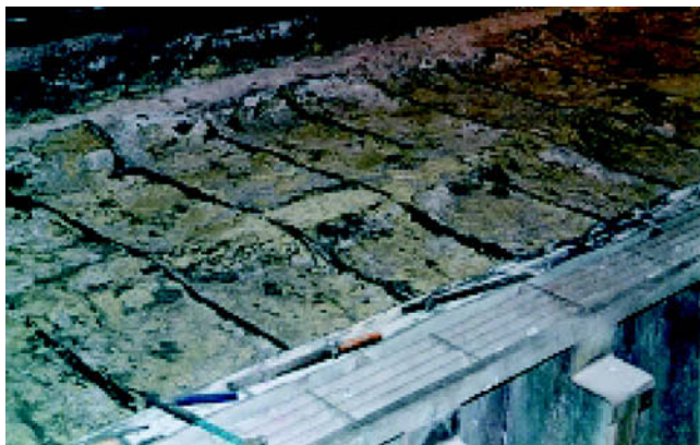
Figure 2: Cleaned surface of the graphite pot before delining.
