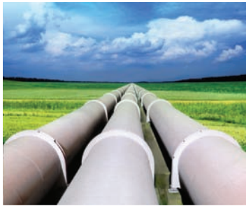
© Sergiy Serdyuk/iStockphoto Polyurethane spheres are used in the maintenance of oil and gas pipelines.
