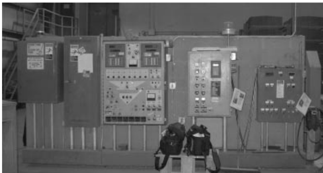
Figure 9.13 A flashing beacon light can be used to alert an operator whether a machine is in automatic or manual mode. The light should be located close to the machine where the operator can see it while attending the machine.
