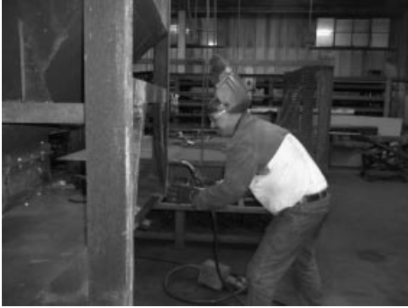
Figure 11.6 A welder using the MIG welding technique.
