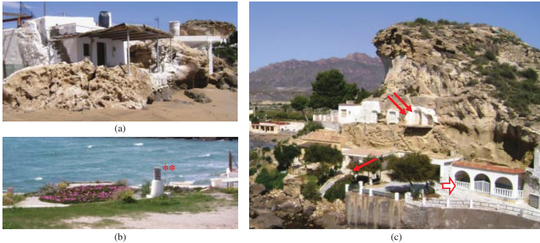
Figure 5.4 The building of cave houses , as opposed to free-standing brick or wood houses, can be viewed as two contrasting construction methods. The first (cave house building) represents a top-down form of construction, where an existing complex 3D structure (the rock cave) is cut out, selectively dug away and simplified down to give the desired shape and function. On the other hand, a free-standing house is fabricated bottom-up, from nothing, using basic building materials of bricks, planks and tiles. The difference is clear in these cave houses in Southern Spain, where (a) is a home built into a rocky outcrop; its chimney (***) and garden (b) show the idea. Larger dwellings are seen in larger rock faces (c), where the entrance (red arrow) and patio (open arrow) might look like a standard house, but the upper windows and balcony (double arrow) give it away.
