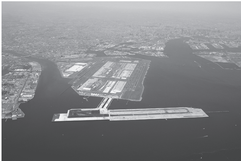
Figure 1.6 Extension of the Tokyo Haneda airport in 2010. (Courtesy of Kanto Regional Development Bureau, Ministry of Land, Infrastructure, Transport and Tourism, Japan.)
