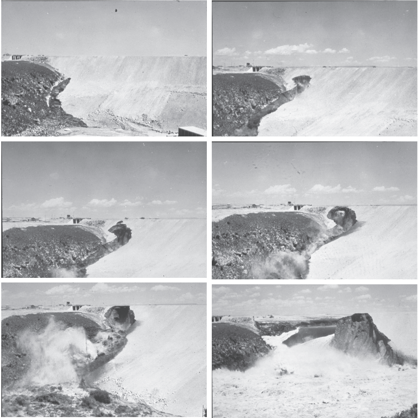
Figure 1.8 Teton Dam seepage failure (1976) (Photos by Mrs. Eunice Olson. Courtesy of Arthur G. Sylvester.)
