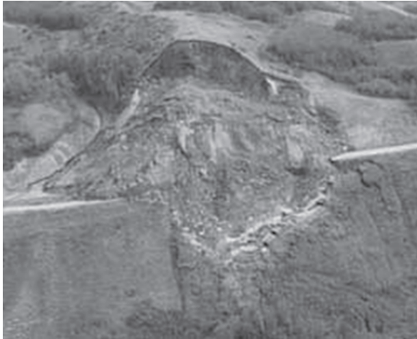
Figure 19.33 Three-dimensional slope failure. (Courtesy of Gordon W. Hunter, British Columbia Ministry of Transportation and Infrastructure.)
