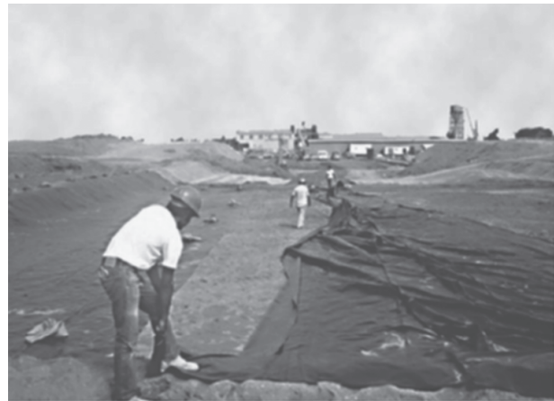
Figure 24.22 Installing a geomembrane in a bottom liner. (Courtesy of Layfield Environmental Systems, Layfield Group Limited, 11120 Silversmith Place, Richmond, British Columbia, Canada V7A 5E4.)
