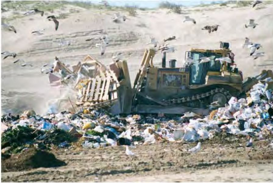
Figure 2. Bulldozer pushing waste from where it is dumped (by waste collection vehicles) to the active landfill face
