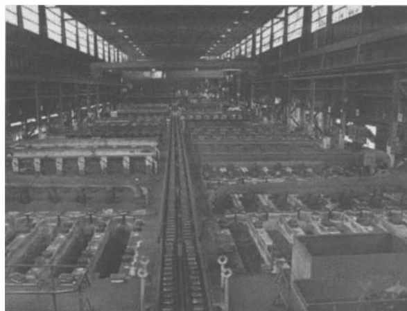
Figure 1 Anode Baking Furnace at Voerdal
