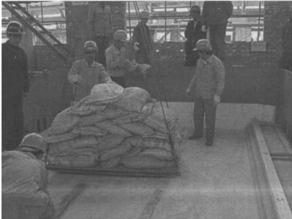
Figure 1: Wooden form for containment of loose DBM
