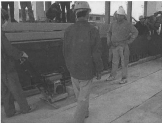
Figure 2: Compaction of DBM using a reciprocating sled
