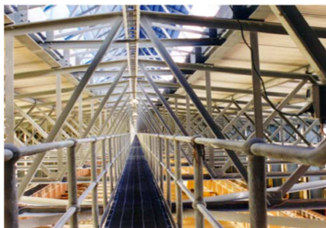
Figure 1: Example of a catwalk under the roofline
