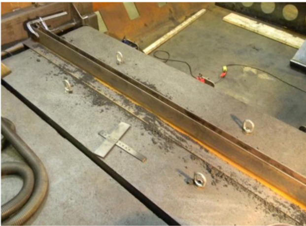
Figure 10. Steel raiser used to make sure that the last layer finishes over the cathodes.
