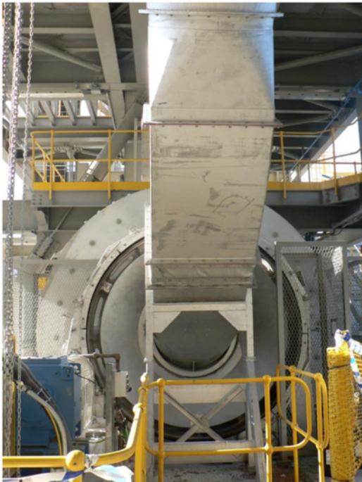
Figure 12 – Air Swept AG Mill Feed end
