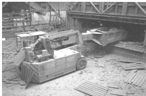
Figure 1: After the explosion in the casthouse.
