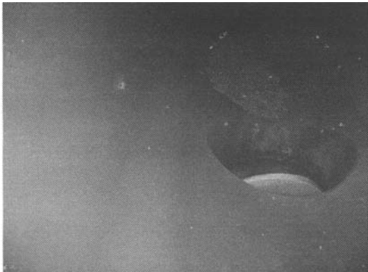
Figure 6: Inside of an Exhaust Ramp after 2 years operation
