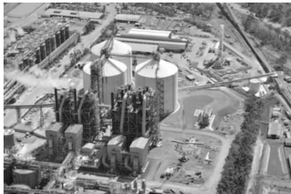
Figure 2. Two (2) x 2300 tpd and Two (2) x 3200 tpd GSC Units at RTA Yarwun, Australia.
