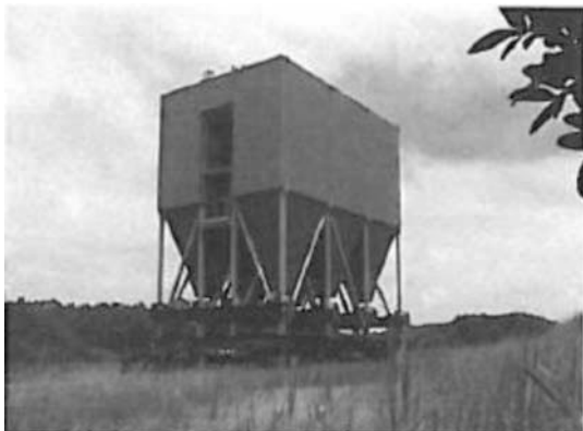
Figure 15. Fabric Filter with 6 m long bags.
