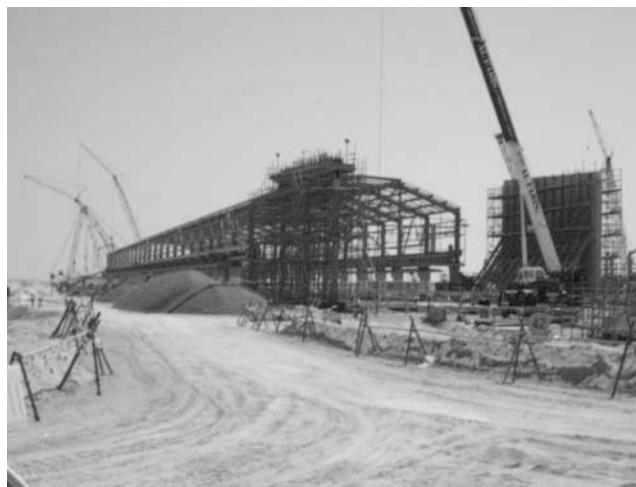
Figure 7. EMAL Phase 2 construction site (October 2012).
