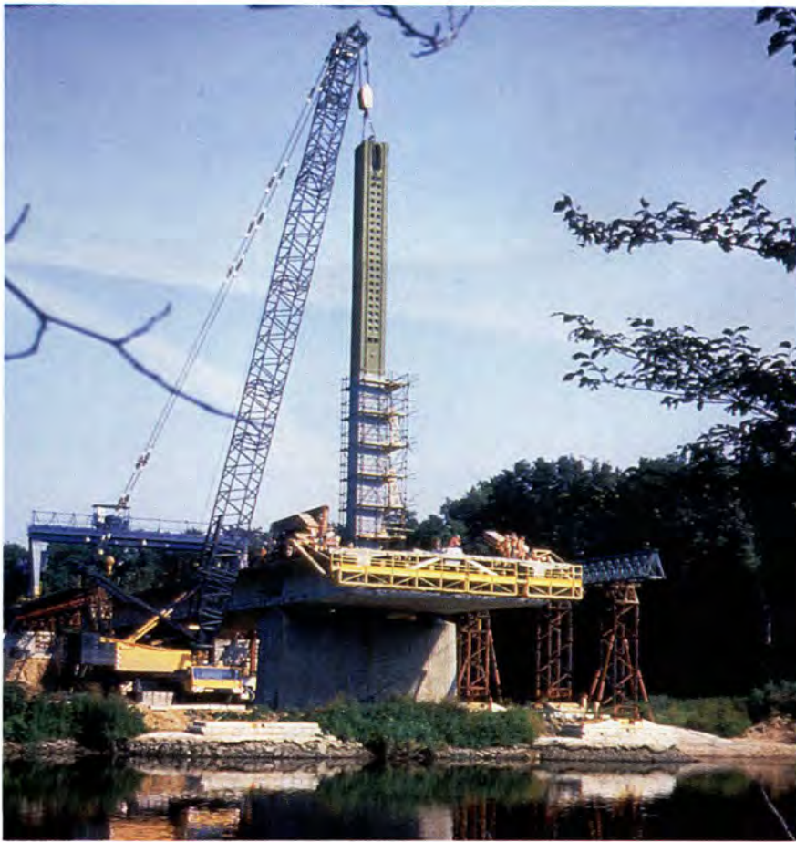
Fig. 21. Elbe River Bridge — erection of the pylon.
