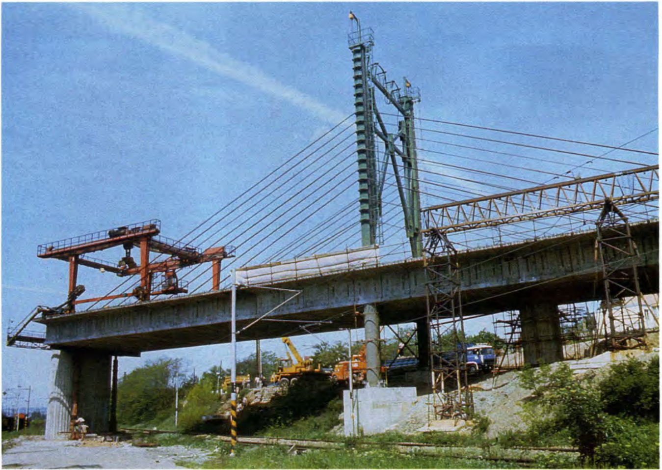
Fig. 36. Vrsovice Bridge — erection of the side spans over the railway.
