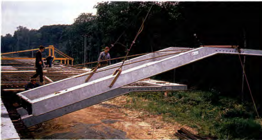
Fig. 17. Elbe River Bridge — typical slab strut.
