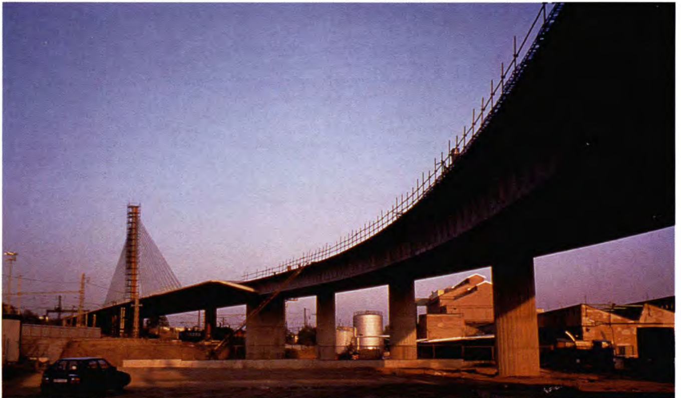
Fig. 40. Vrsovice Bridge — progressive assembly of the deck.
