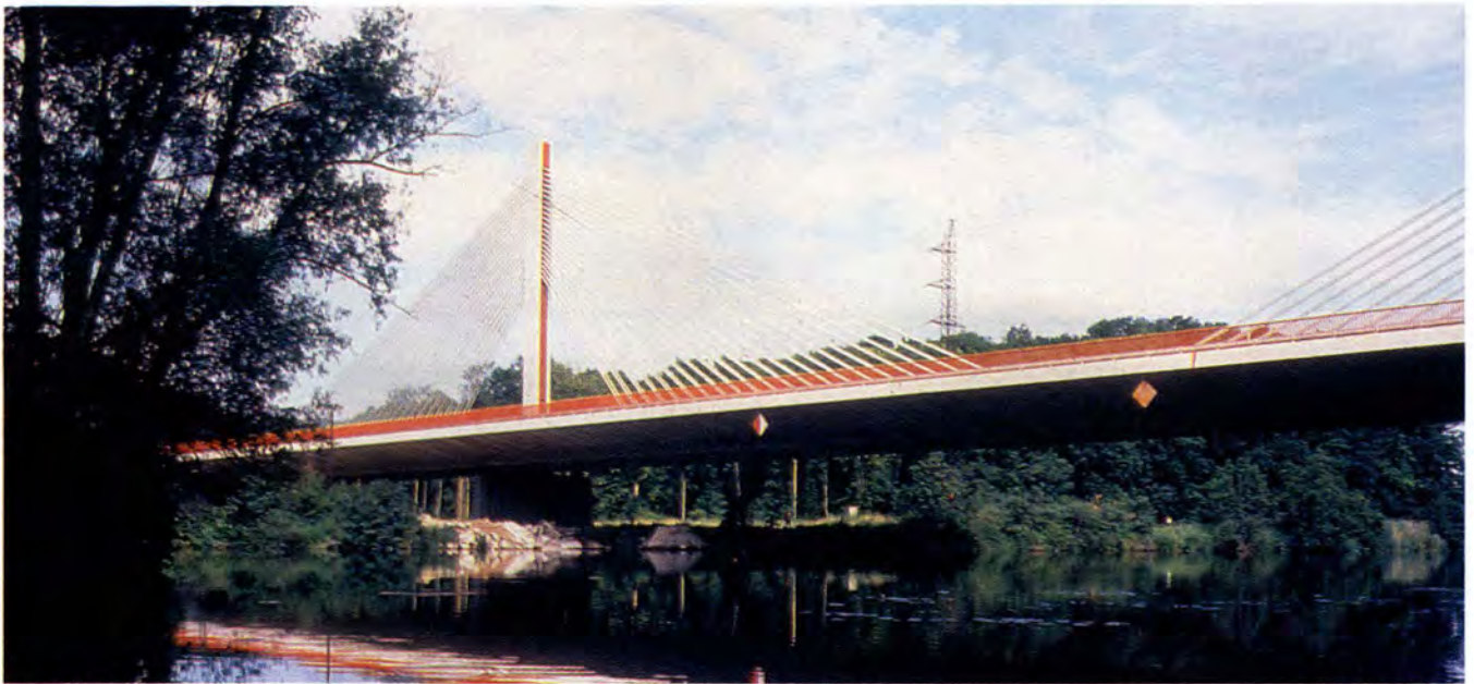
Fig. 1. Elbe River Bridge.
