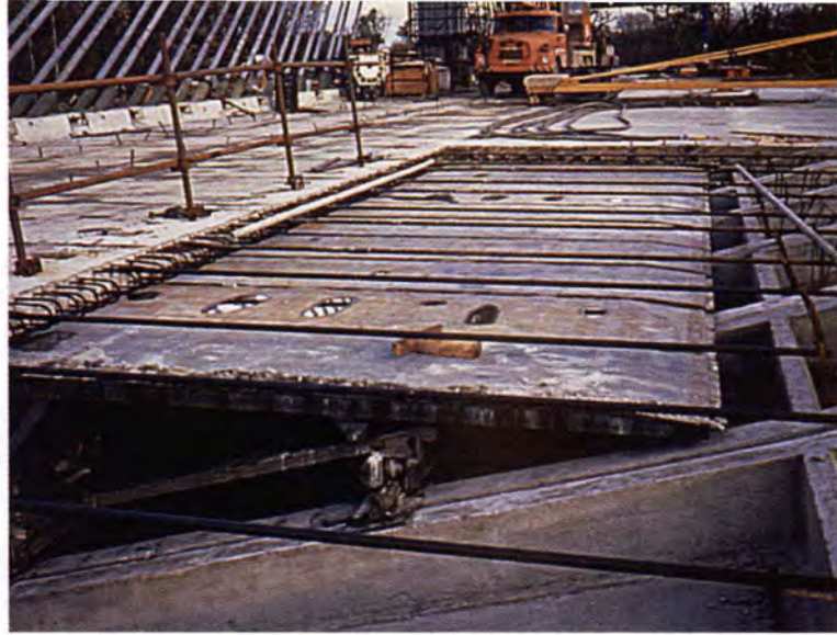
Fig. 32. Elbe River Bridge — movable formwork for casting of the deck slab.
