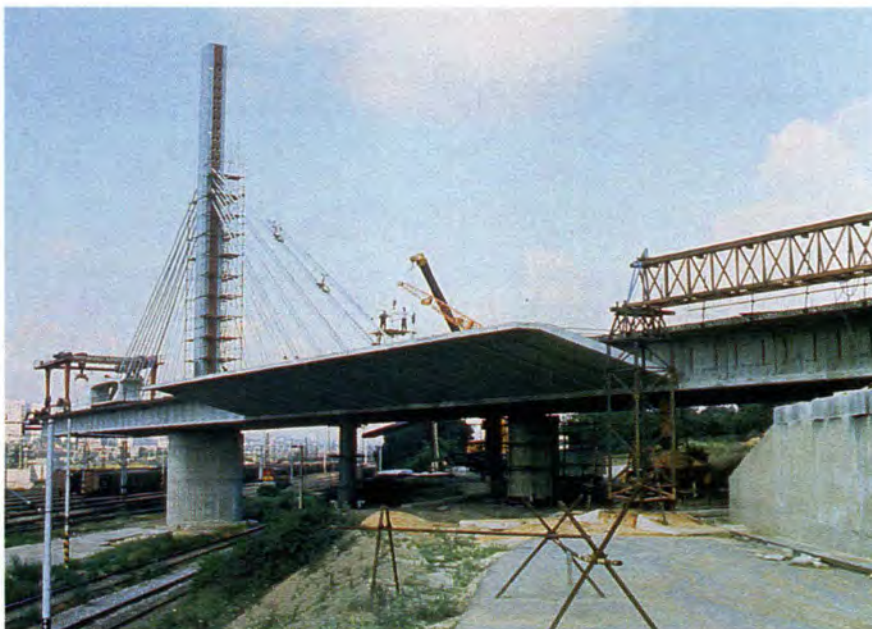
Fig. 37. Vrsovice Bridge — erection of the main span.
