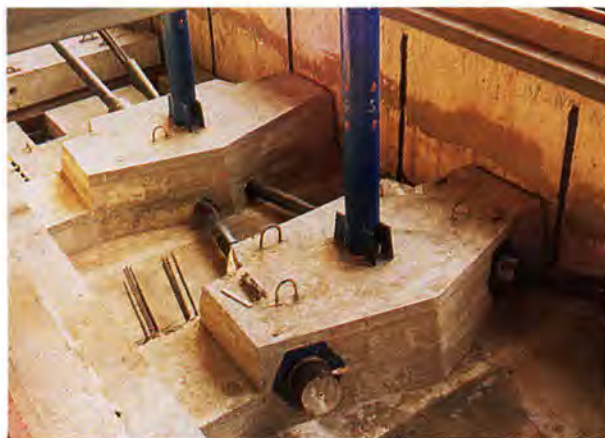
Fig. 19. Vrsovice Bridge — testing of the external cables.
