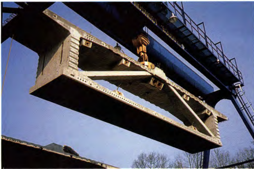
Fig. 13. Elbe River Bridge — typical segment.
