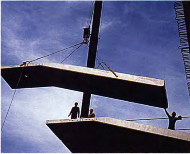
Fig. 31. Elbe River Bridge — erection of a precast slab strut.
