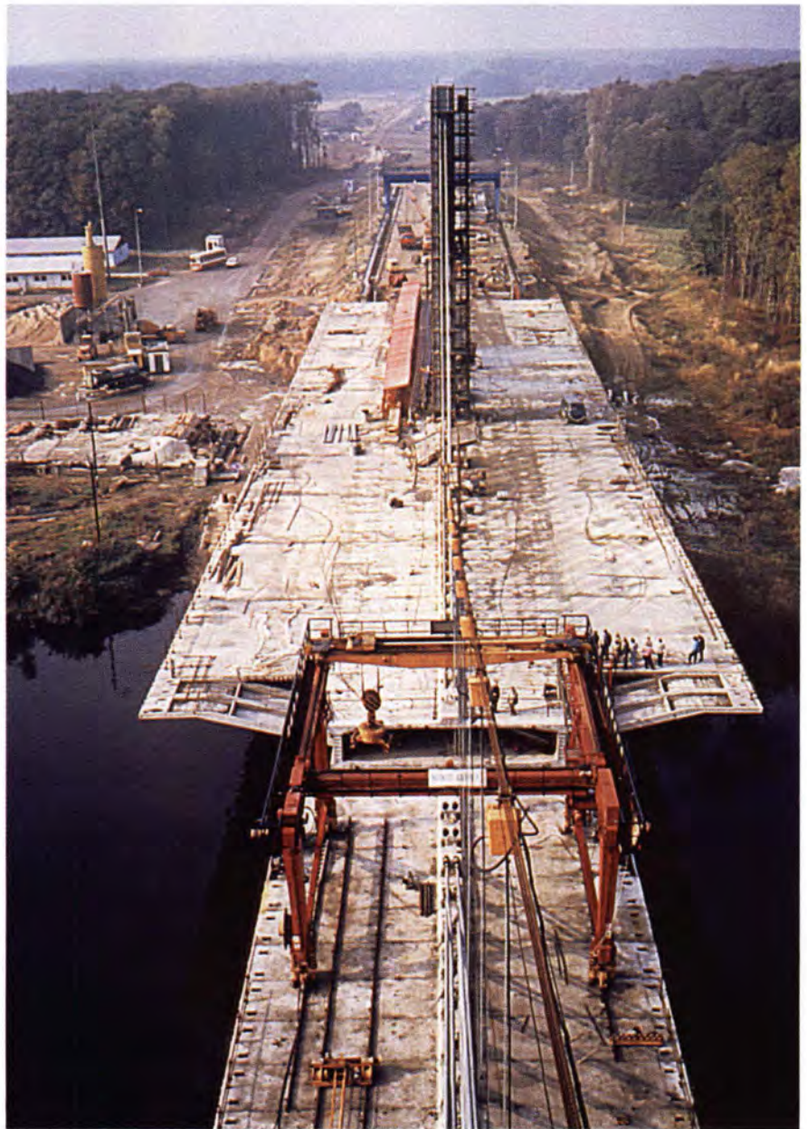
Fig. 33. Elbe River Bridge — progressive assembly of the deck.
