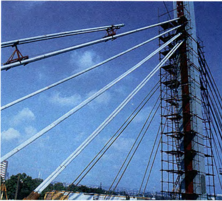
Fig. 38. Vrsovice Bridge — erection of steel tubes of the stay cables.
