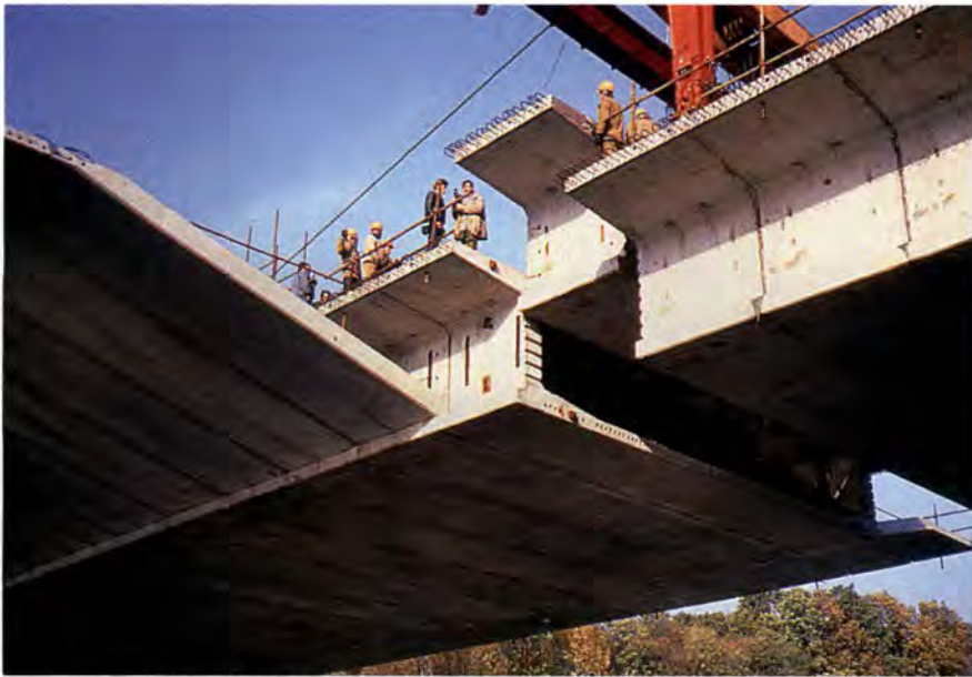
Fig. 34. Elbe River Bridge — erection of the closure segment.
