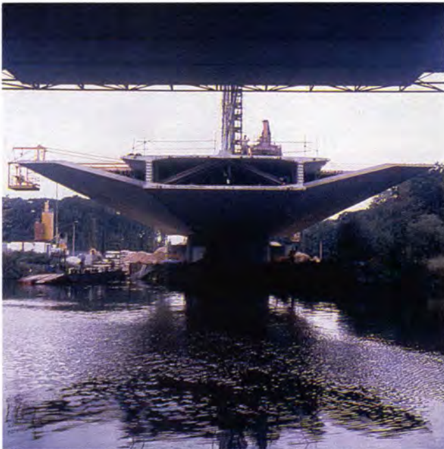
Fig. 4. Elbe River Bridge — deck.
