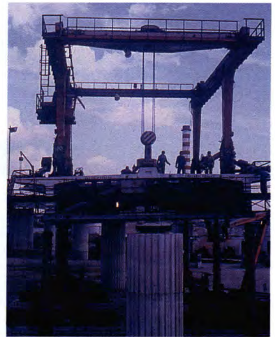
Fig. 39. Vrsovice Bridge — erection of a segment of the approach spans.
