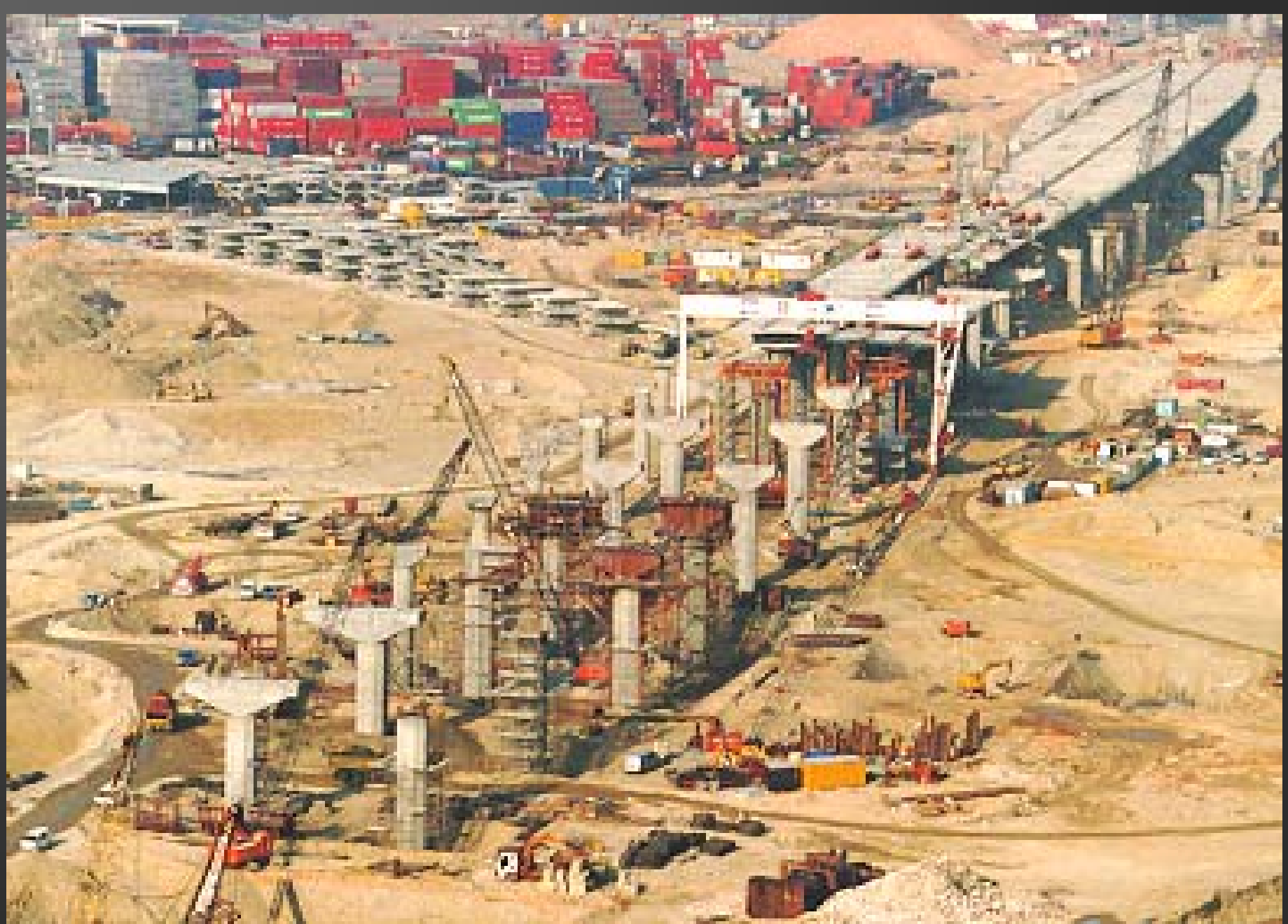
Forming the elevated bridge of the West Kowloon Expressway
