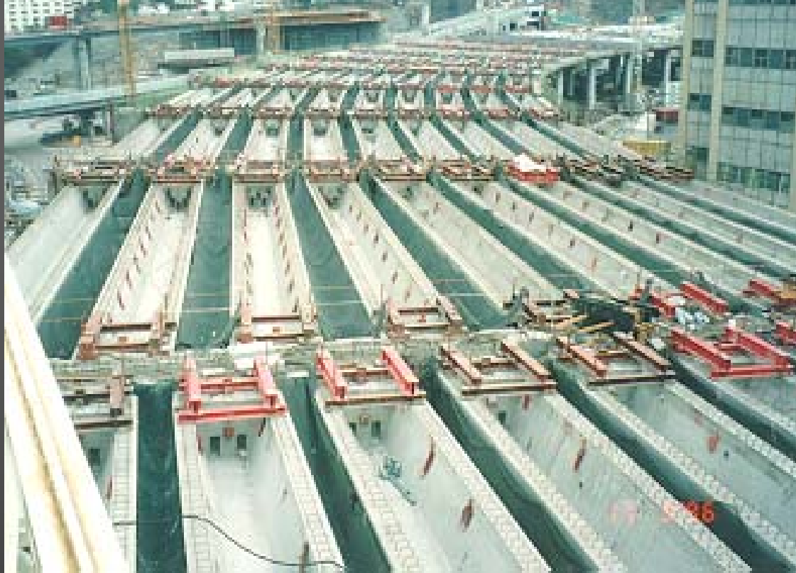
Precast V-shape beam for the Route 3 elevated expressway at Kwai Chung
