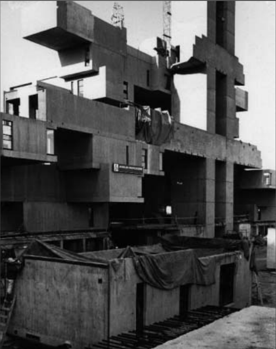
Installation of the modulated units and the associated structure
