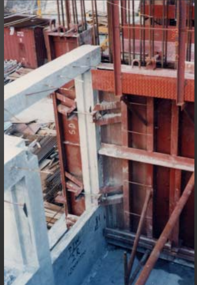
Detail of façade installation using in-situ jointing arrangement in the later version of Harmony Block Construction
