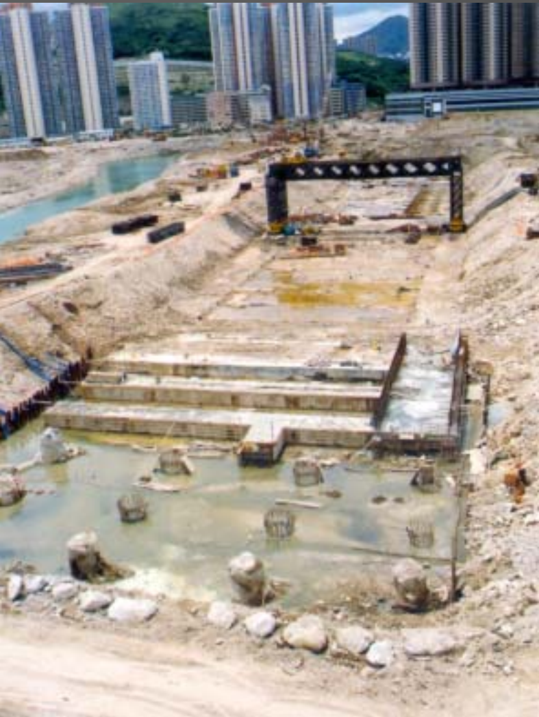
Prepare for the foundation to support the culvert
