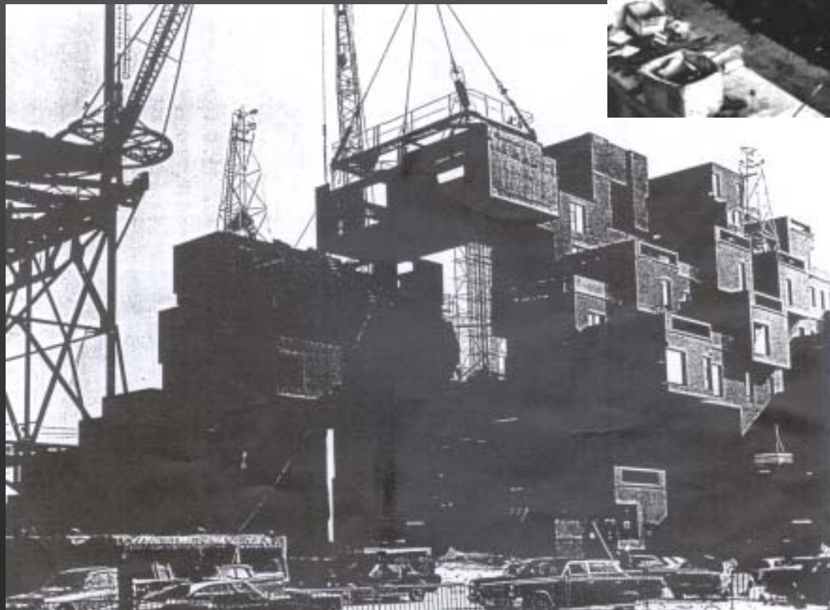
Forming and Installation of the modulated units
