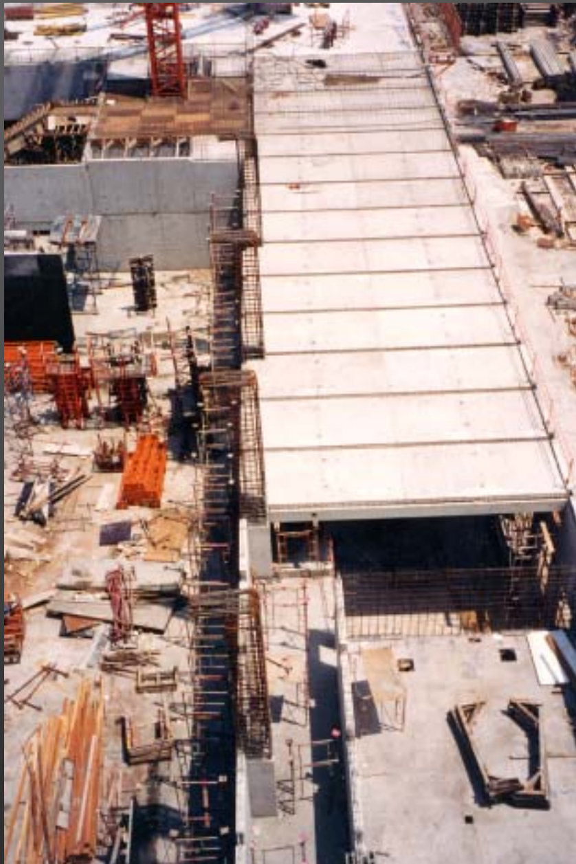
Forming the floor slab using precast secondary beams and semi-slab for the main building (above) and members' complex (right)
