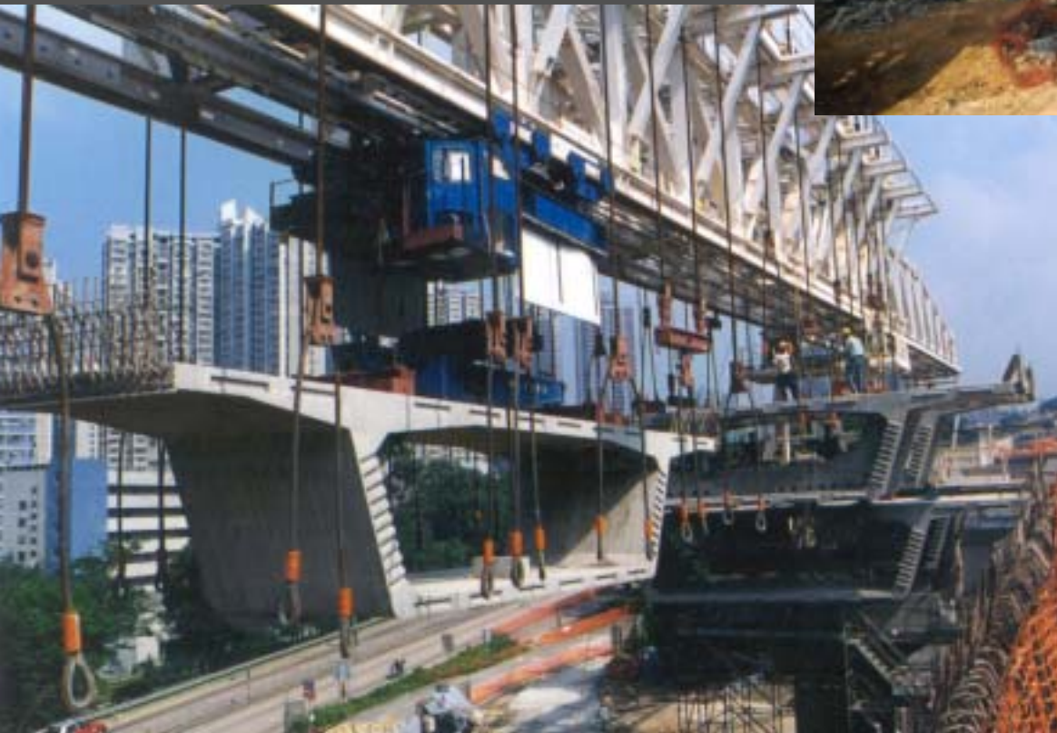
Installation of the box-girders
