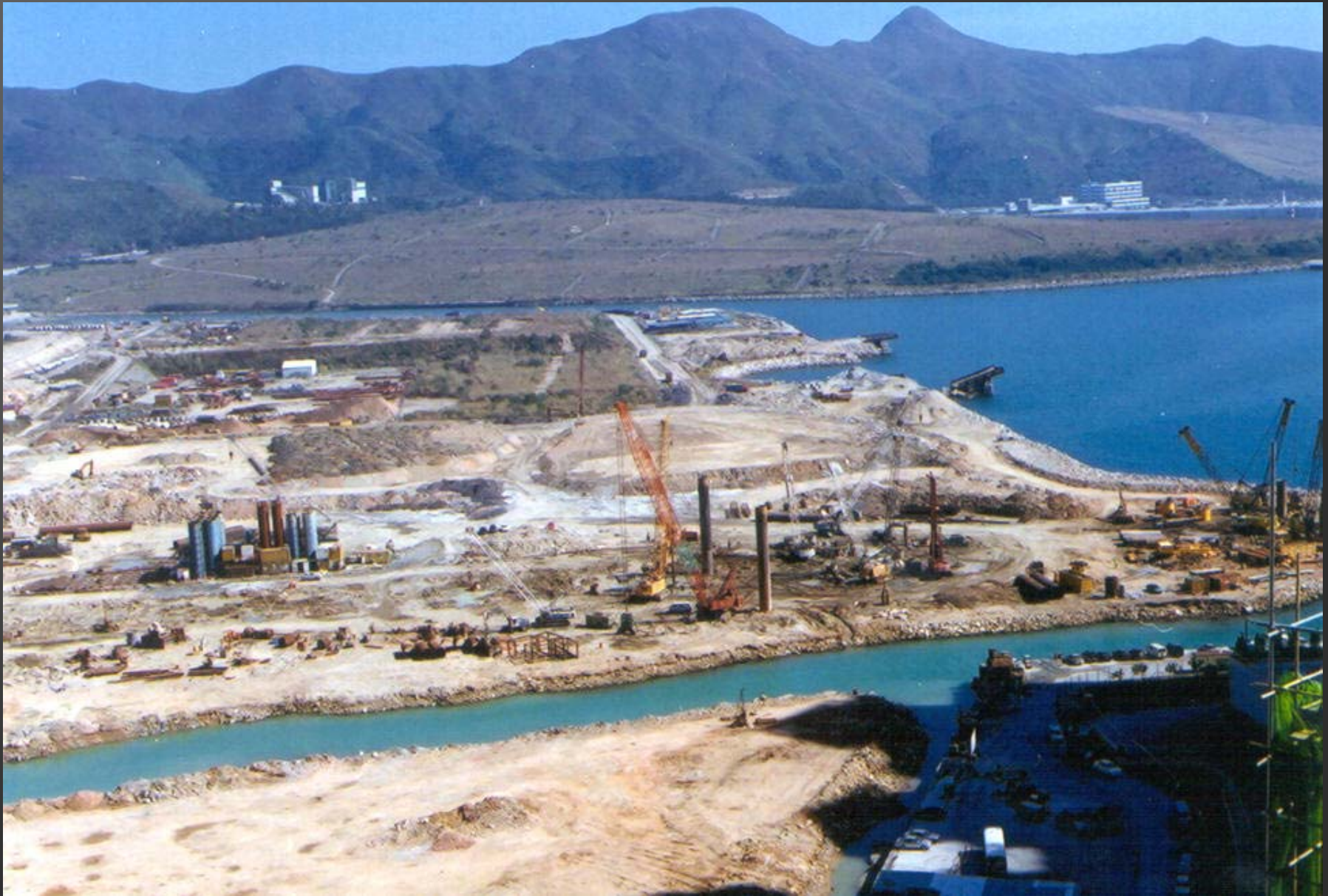
Forming storm water discharge culvert – Tseung Kwan O Reclamation
