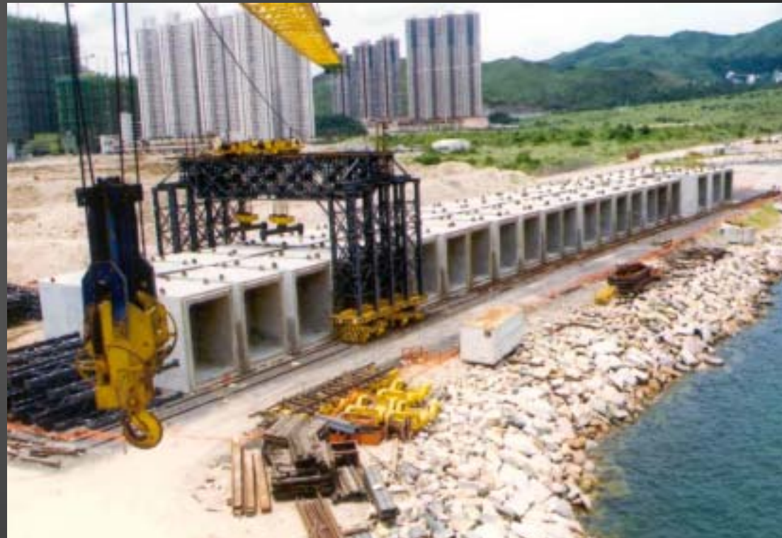
Delivery and storage along the temporary seawall
