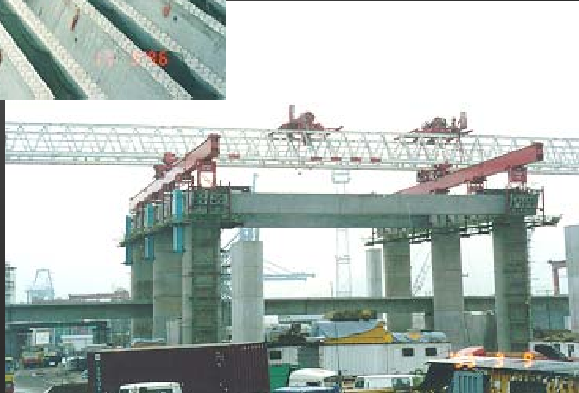
Precast V-shape beam being lifted to pier head by launching gantry
