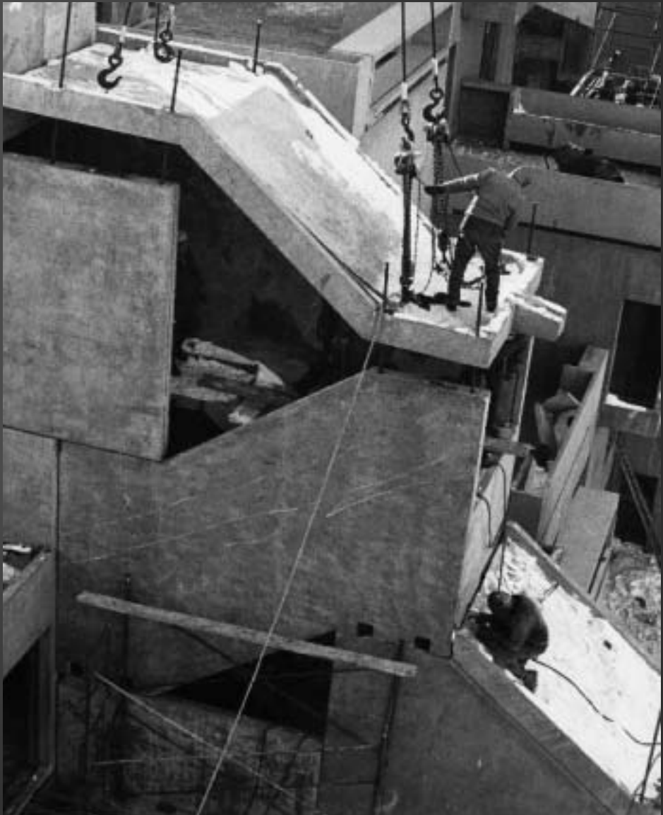
Installation of the modulated units and the associated structure
