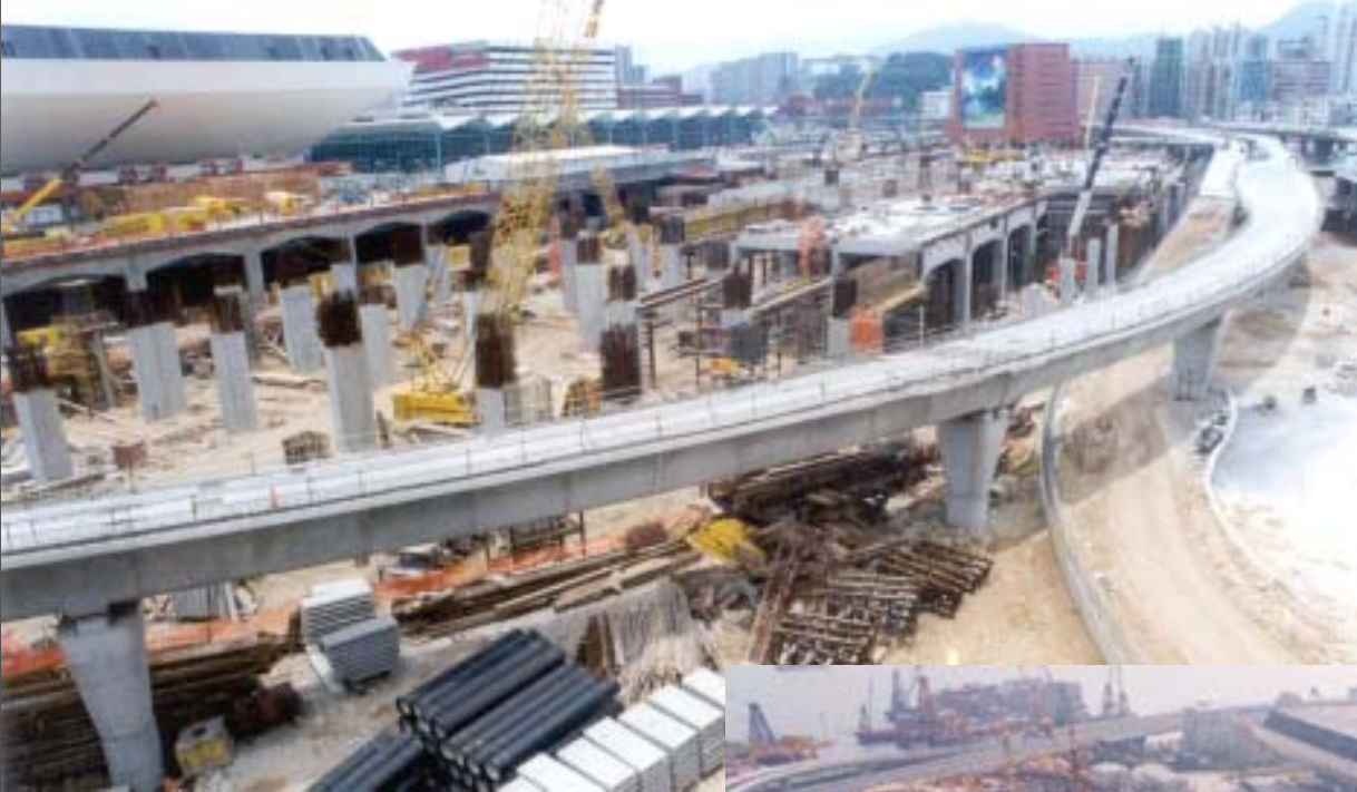
Kowloon Canton Railway Station podium/deck
